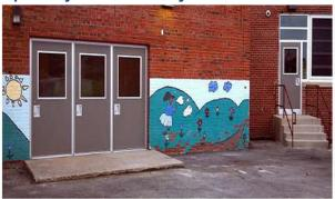
Forced Entry Bullet Resistant TASKDOOR prevents ballistic and forced-entry attack. The door is equipped with advanced materials that provide an elevated threat protection solution to withstand 15 minutes of simulated "mob" attack and resistant to ballistic rounds. Forced Entry Bullet Resistant Assemblies safeguard anywhere where the highest level of protection and durability are important considerations.
